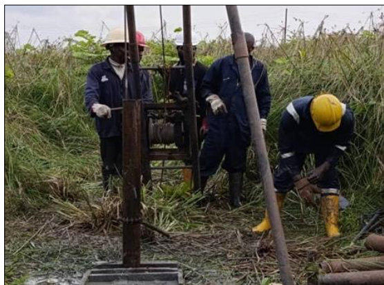
Figure 9 A boring activity with a manual drilling rig
